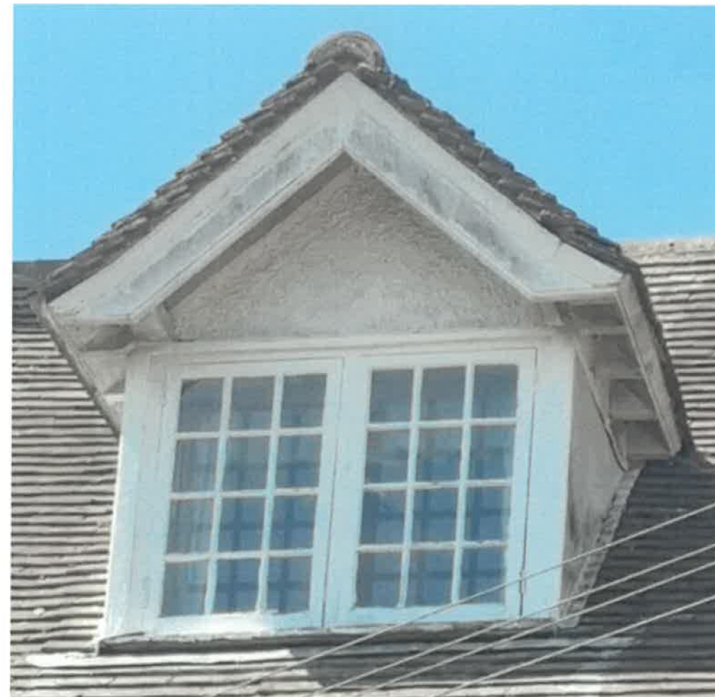
Photo of existing dormer (WS2, WS3 & WS4 are the same)
