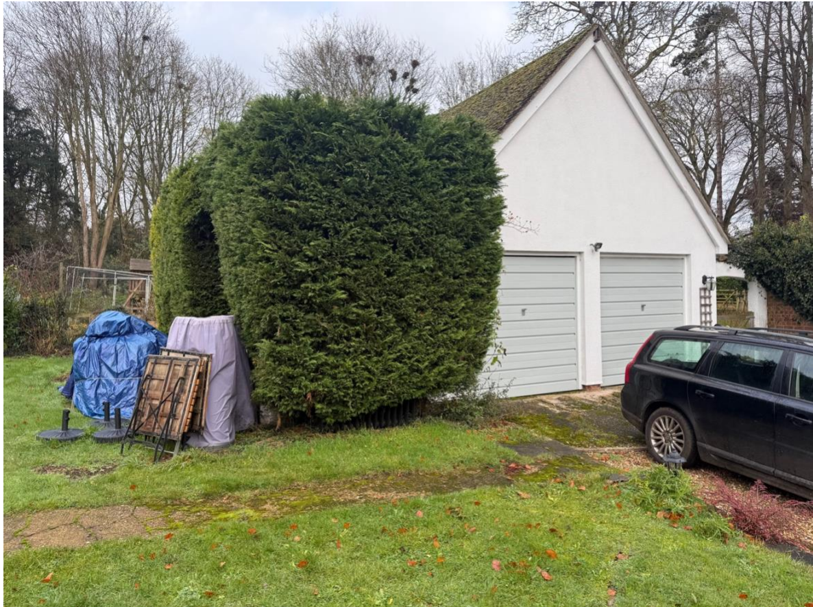
Figure 3-6 South face of the double garage showing leylandii concealing oil tank
