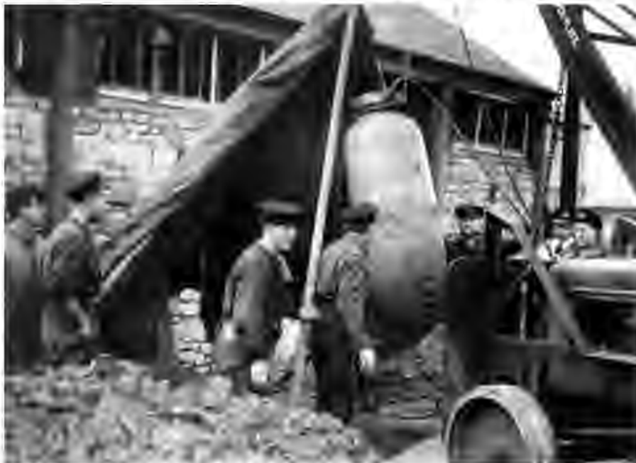
Removal of an UXB
