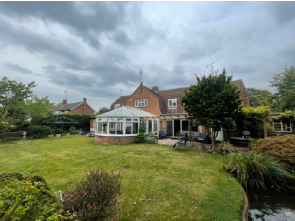
6. Rear elevation viewed from garden. The non-original conservatory and windows will be removed, with Crittall-style frames replicating the original fittings installed to all openings
