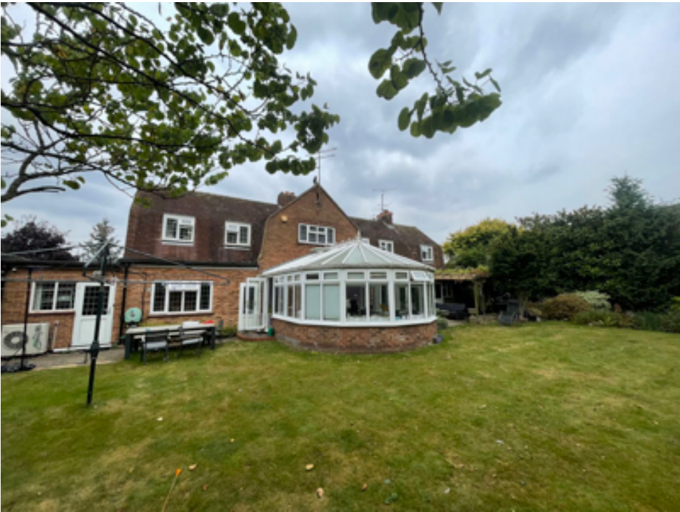
5. Rear elevation showing uPVC conservatory and windows to be removed
