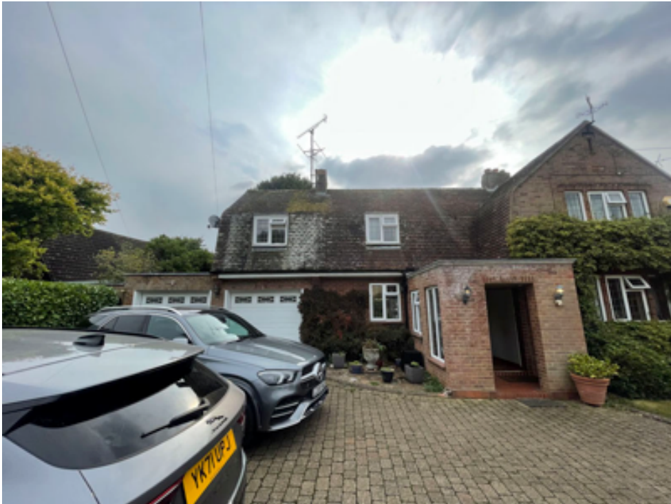
1. Front elevation showing window to left of porch that we propose to enlarge
