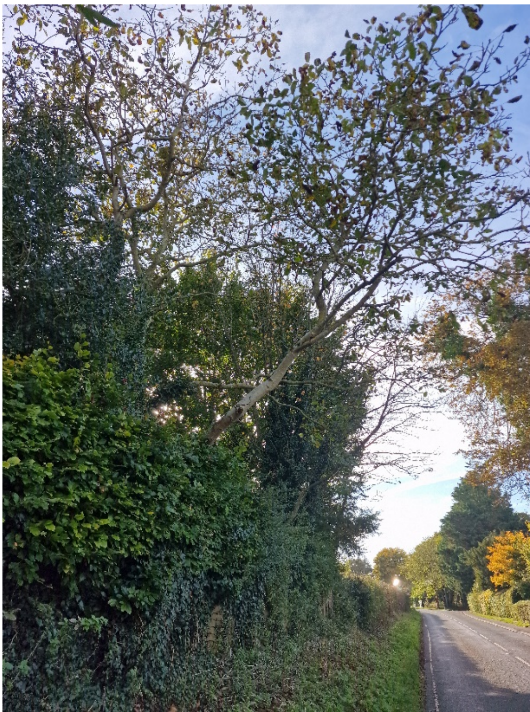
View looking south . The 'lean' on one of the boles can be easily seen. I am concerned this will fall in the road
