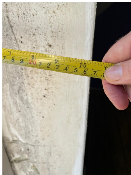
Picture 2 – Wall thickness demonstrated.
