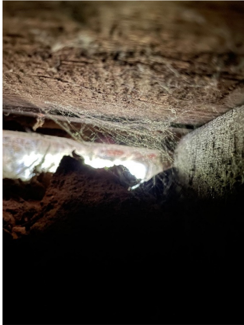
Picture 3 and 4 – Ventilation and clearly ventilated void.
