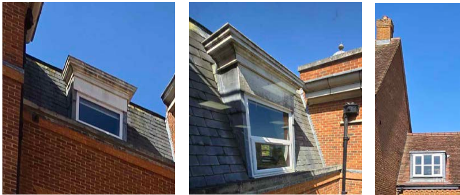
FIGURE 11: EXISTING DORMERS AT THE PRIORY AND SURROUNDING
