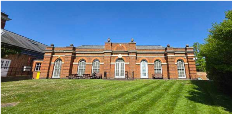
6 Ancillary Building B: South west elevation
