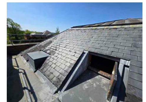
9 Roof and access door
