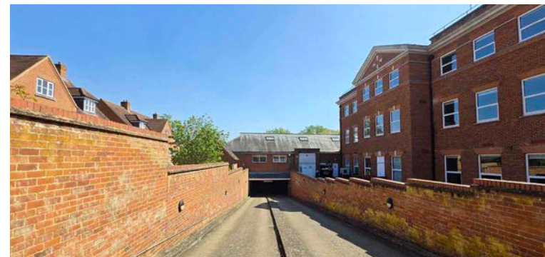
5 Basement access ramp
