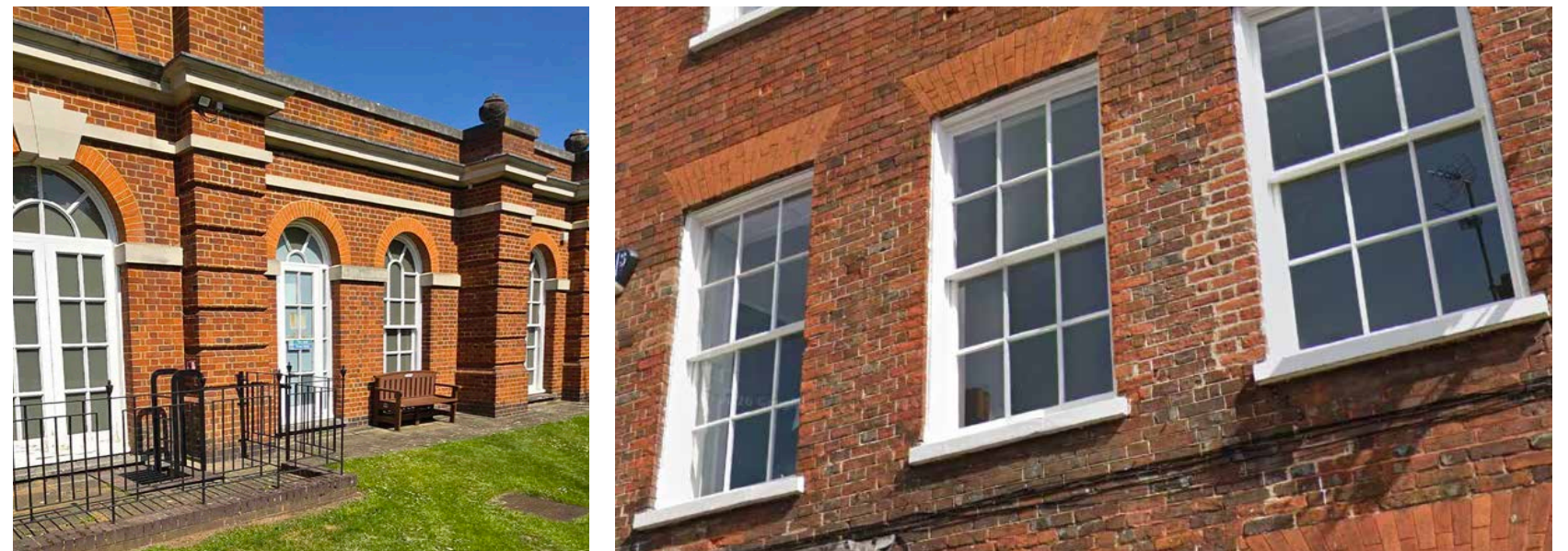
FIGURE 15: EXISTING WINDOWS WITH WINDOW BARS AT THE PRIORY AND IN LOCAL AREA
