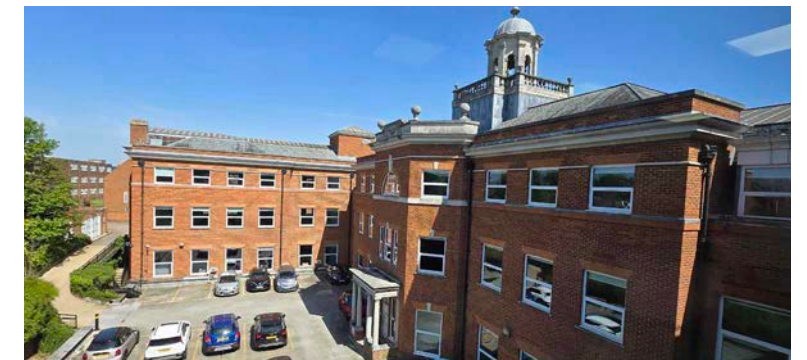
6 Rear parking court
