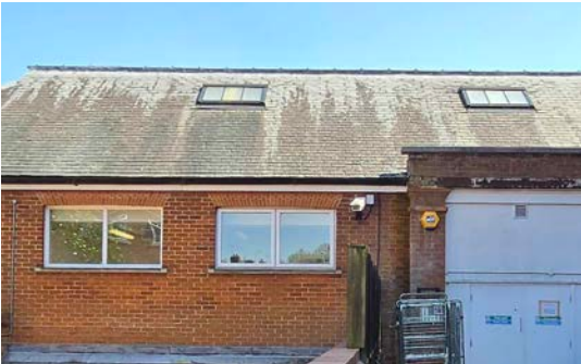
FIGURE 19: EXISTING ROOF WINDOWS
