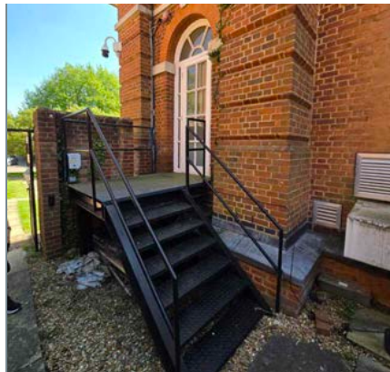
8 Ancillary Building B: Stepped access to building
