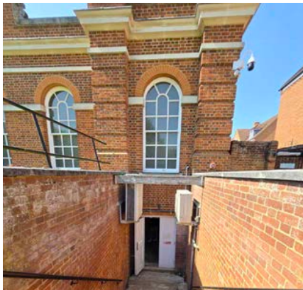
7 Ancillary Building B: Stepped access to basement
