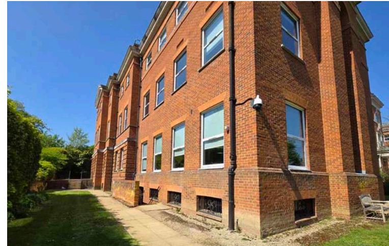
3 South east / west elevation, building corner
