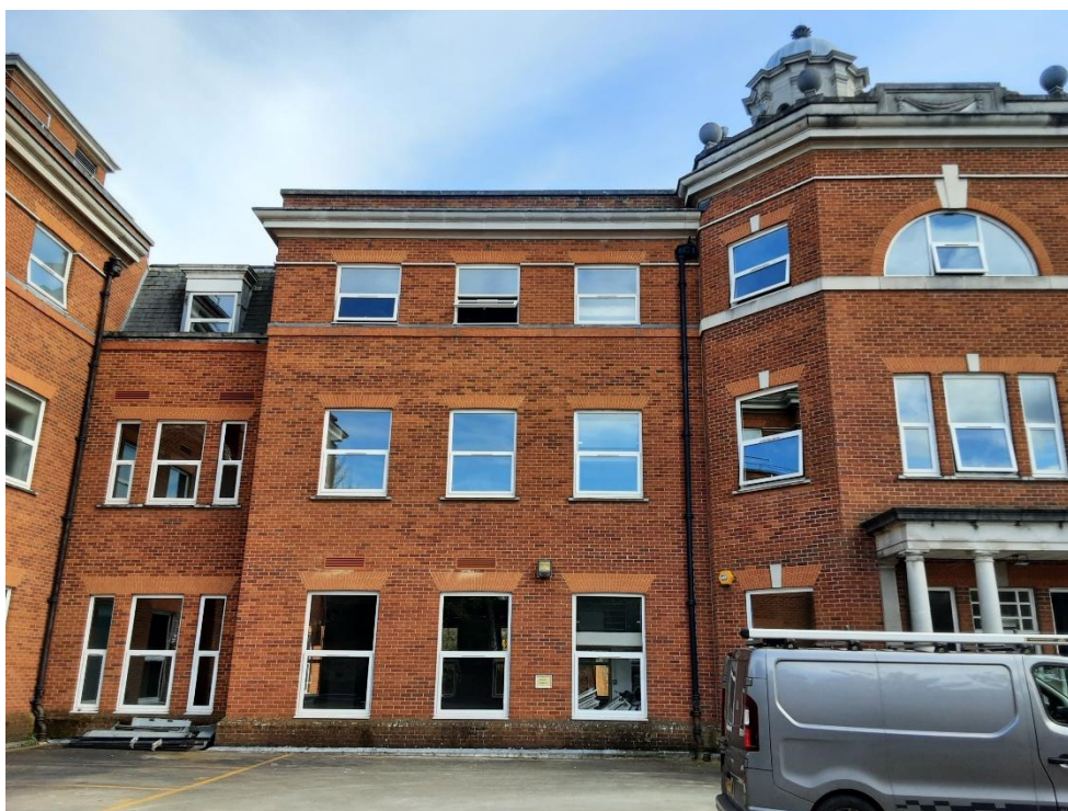
Photograph 2: Buildings: Radcliffe House
