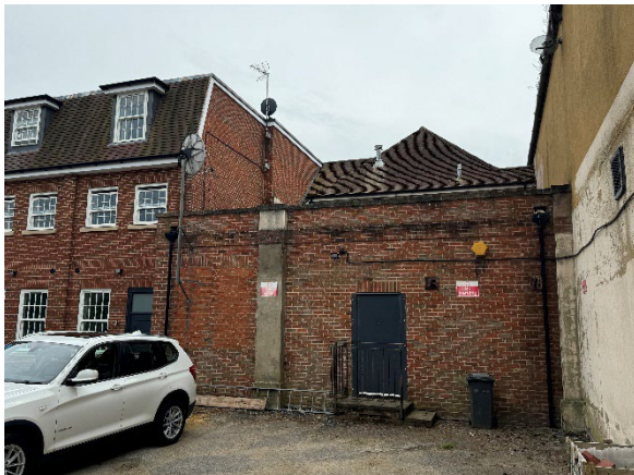
Rear yard and adjacent building at 8-10
