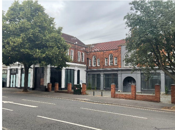
View from south east towards site
