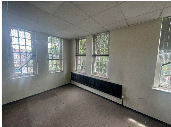
Internal view at first floor level
