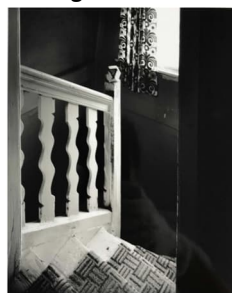
Figure 4.14: 1992-94 photograph showing the historic splat balusters and newel post in the stair wing (Source: Historic England Archives, Reference: BBS2/06134).
