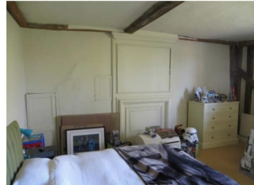
Figure 4.150: Showing the western wall of the north-eastern bedroom.
