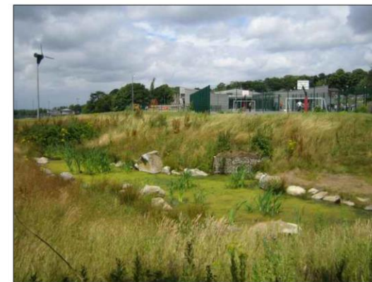
Above: Examples of attenuation basins both when wet and dry, the marginal planting of wetland species will increase the biodiversity on site
