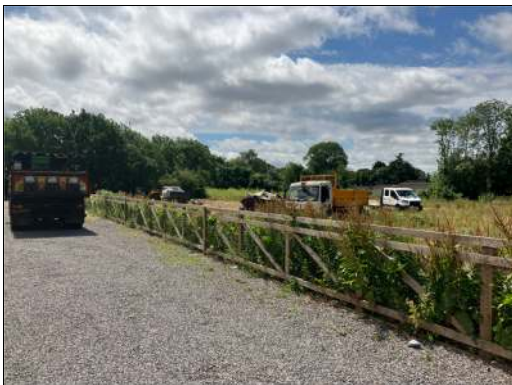
Photograph 5: Dividing fence in central north of site, view south east.
