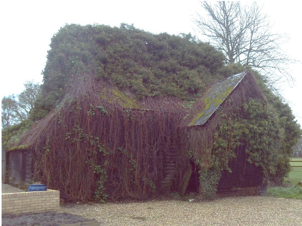
Plate 2: Exterior view of barn covered in common ivy
