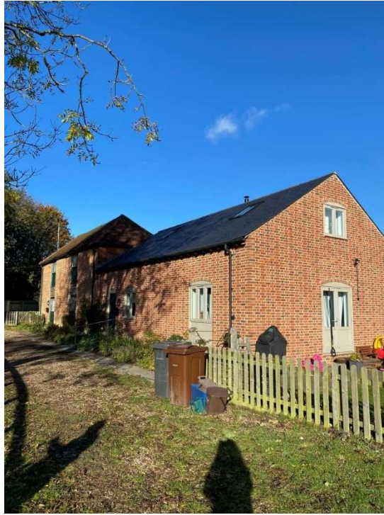
Image of No. 18 on the north side of the courtyard
