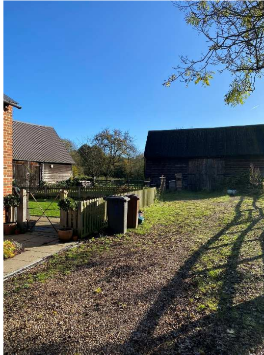
Image of eastern barn and the listed barn as seen from the north west of the proposed site across the courtyard
