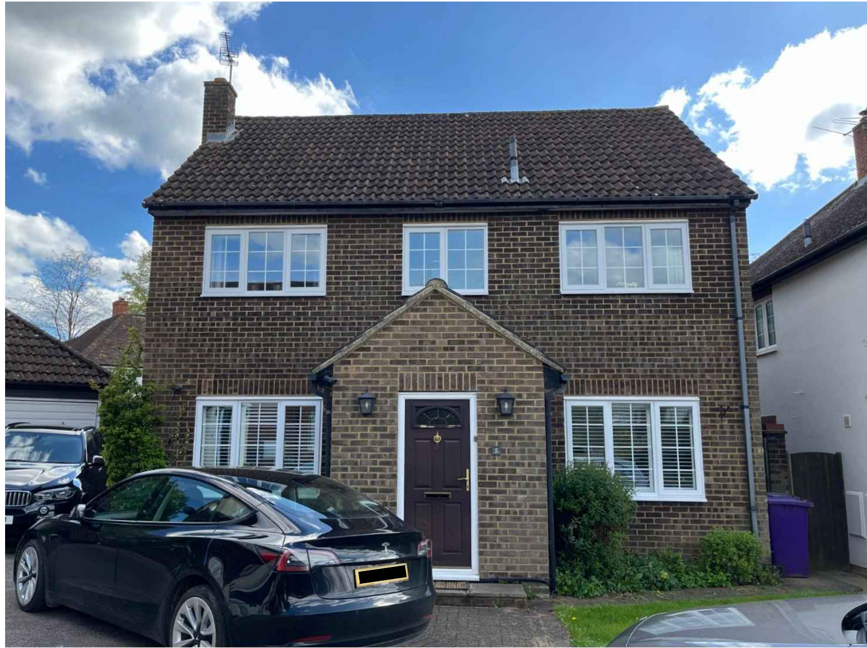
FRONT VIEW OF EXISTING PROPERTY
