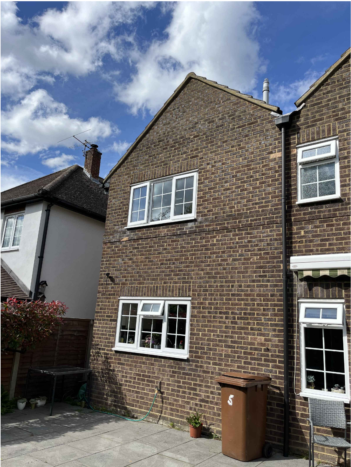
REAR VIEW OF EXISTING PROPERTY
