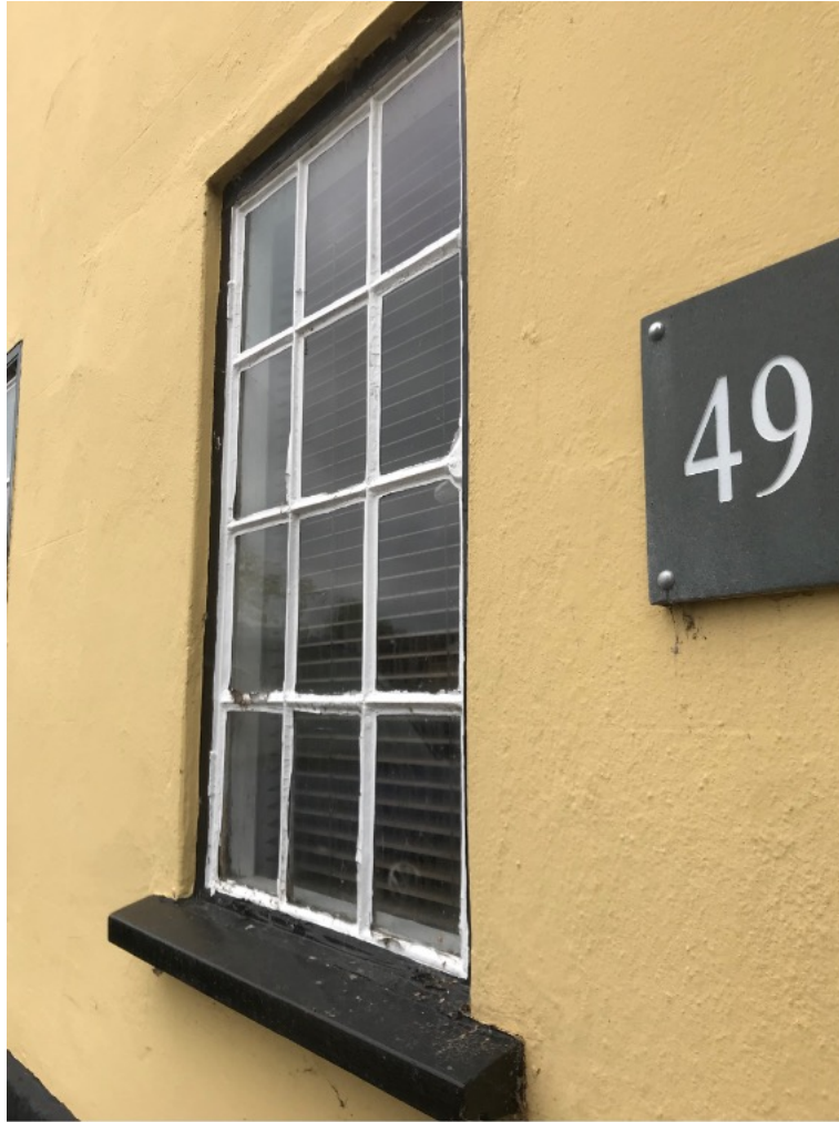
Picture 6: Single casement ground floor entrance hall, external (plastic sill)
