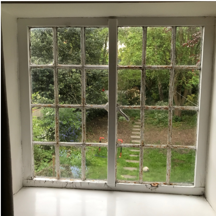
Picture 19: First floor main bedroom double casement, internal
