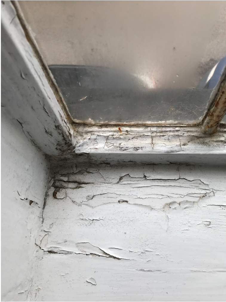
Picture 12: Double casement first floor bathroom window corner
