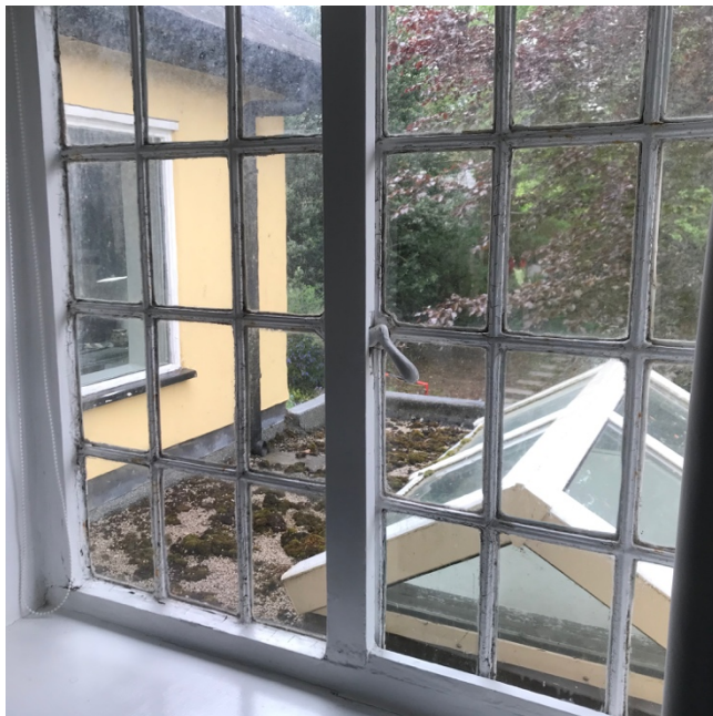
Picture 15: First floor double casement window rear bedroom
