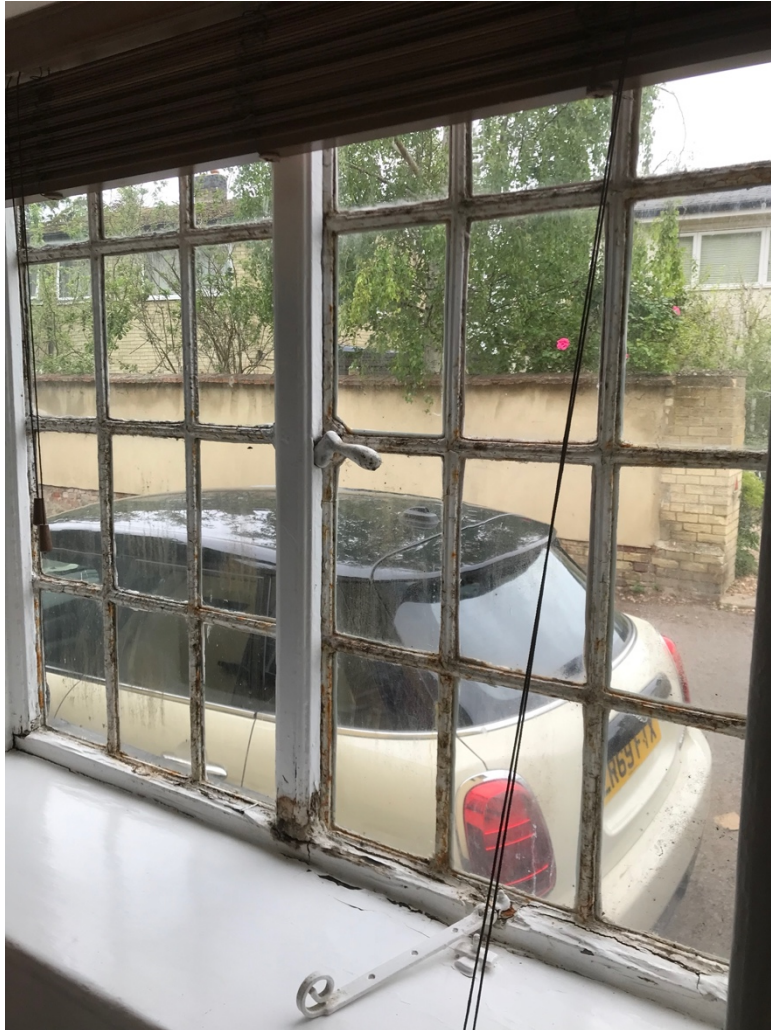
Picture 8 and 9: Double casement ground floor entrance hall, internal (painted shut)
