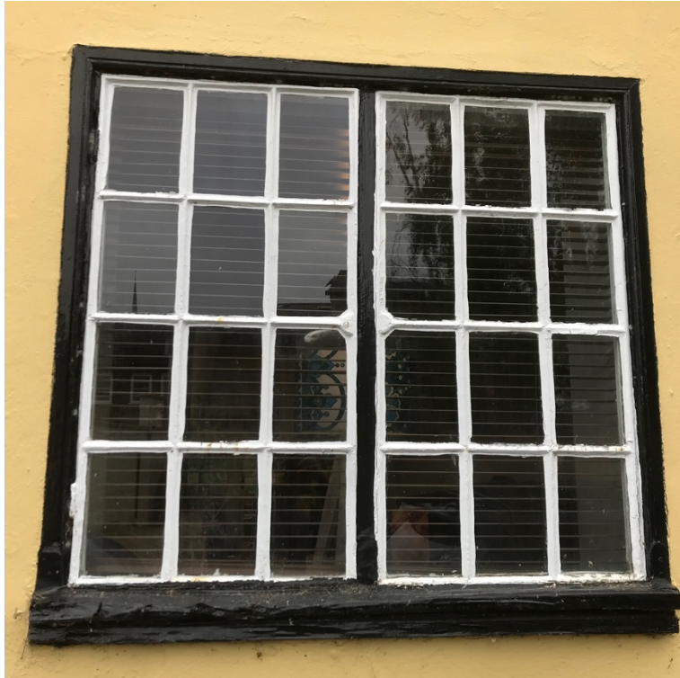
Picture 4 & 5: Double casement ground floor entrance hall, external
