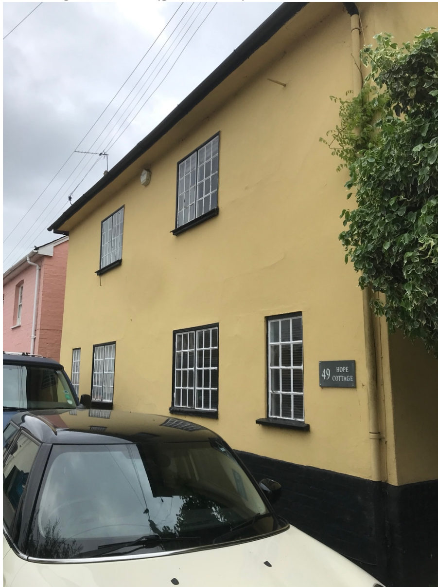
Picture 7: Front of house showing 4 double casement (two first floor, two ground floor), and 2 single casement (ground floor) windows
