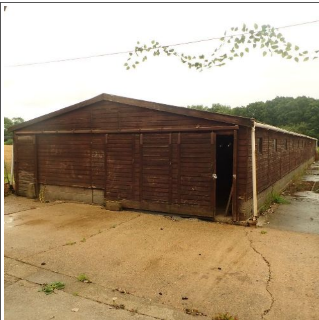
Figure 13: Building 3 - western end
