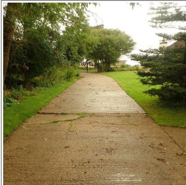
Figure 21: Entrance road to yard
