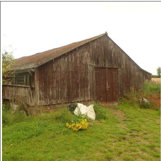
Figure 16: Building 5: eastern gable
