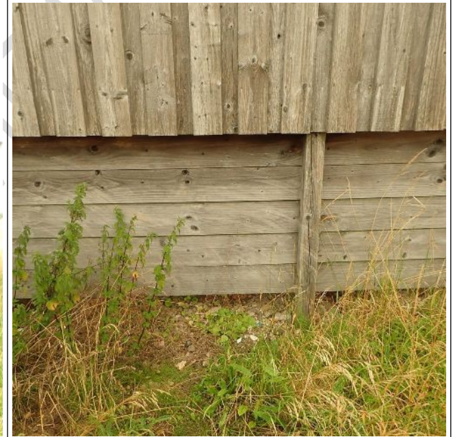
Figure 9: Building 1 - southern wall
