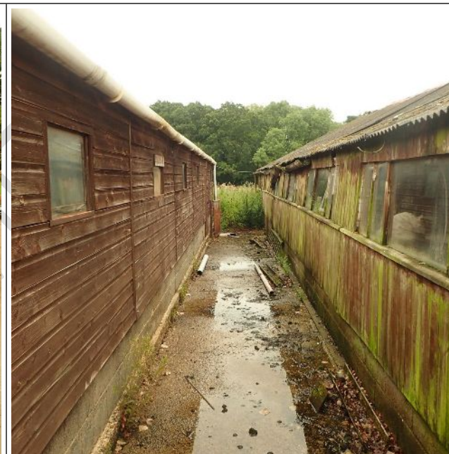
Figure 15: Building 2 to left with Building 5 to right
