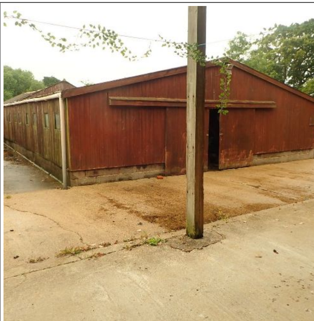
Figure 14: Building 4 - western gable
