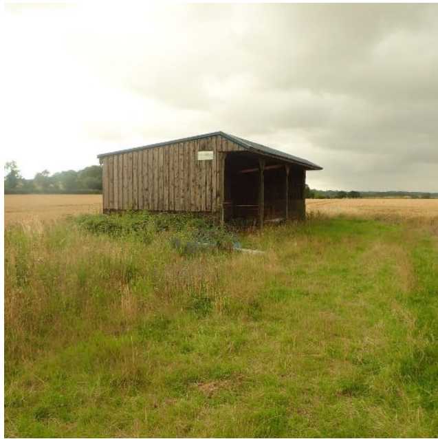
Figure 7: Building 1 - view from east
