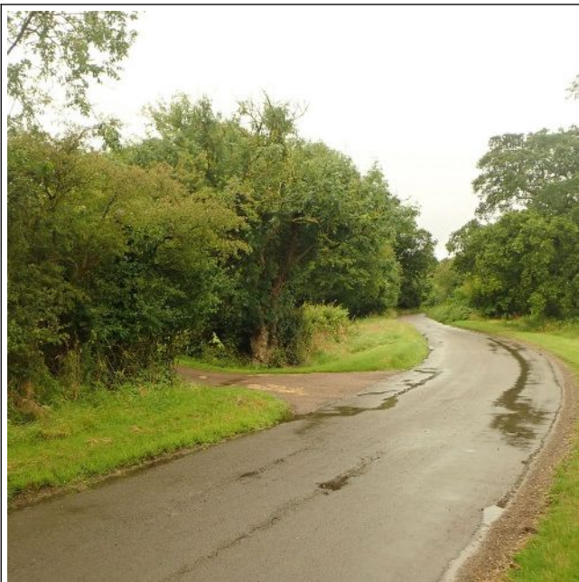
Figure 23: Main road looking north with entrance to Building 1 on left
