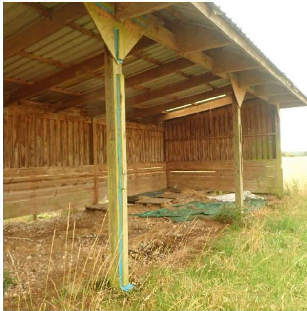
Figure 8: Building 1 - open north side
