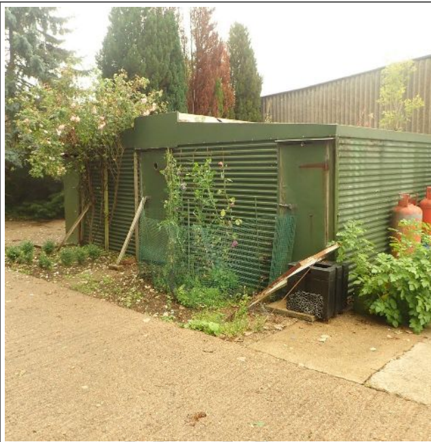
Figure 20: Building 7 from south side with Building 2 behind
