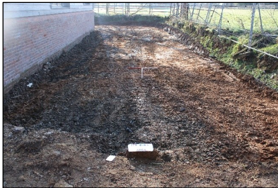
Plate 7: Stripped area, western part, looking SSE
