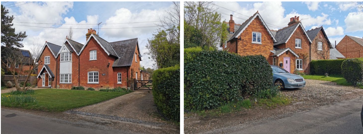
Figure 2: Photographs of Lagonda Stud and Sunnyside Cottage, at the site's frontage, facing Pottersheath Road
