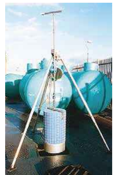
Step 9 – Once the coalescer unit is above ground level, swing it to one side of the manhole for maintenance.
