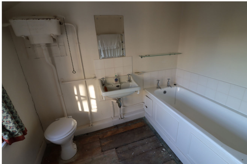
Image6 : partition on right (C20th) to be removed and this will become a larger Cottage bathroom.
