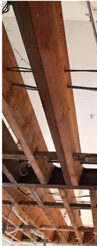
Image 2. Kitchen ceiling joists and the steel to be removed – Clearly showing they are C20th
