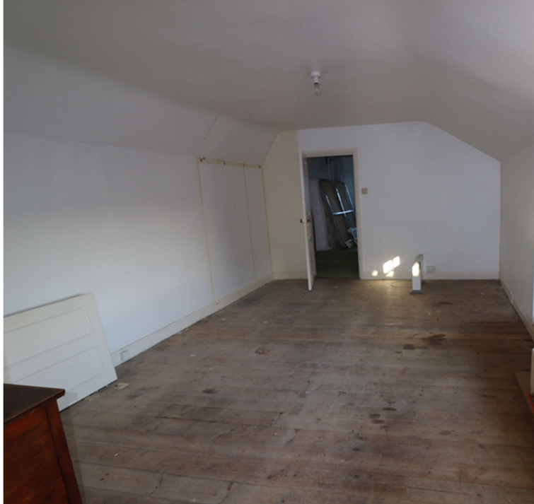
Image 3: Looking East in the room above the Kitchen – Blockwork wall on the left is to be removed and the C20th partition at the end removed and rebuilt slightly further back on the Kitchen beam line below.
