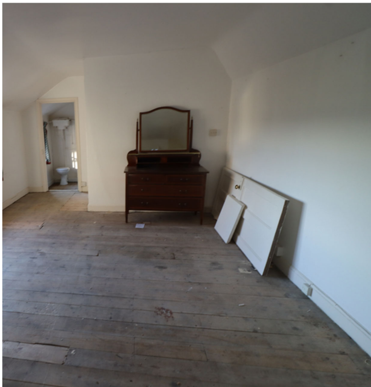
Image 4: Looking West toward chimney stack in the room above the Kitchen – door on left to be infilled and C20th Blockwork wall on right removed
