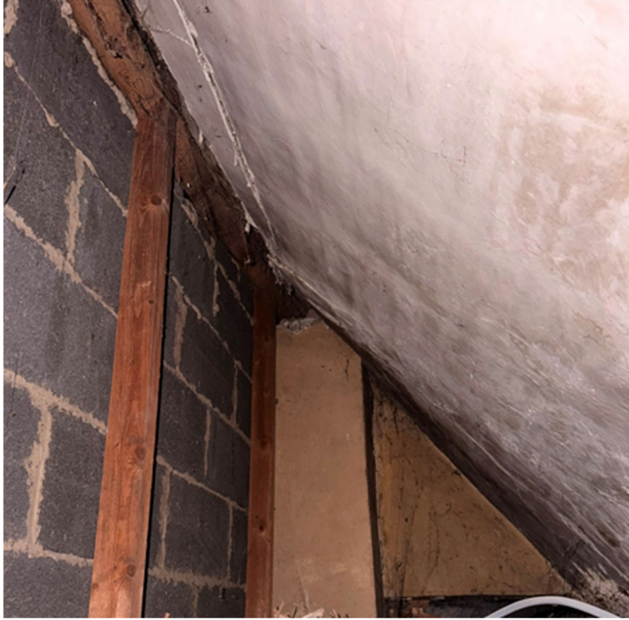
Image 5: The C20 block wall to be removed on the North side of the room above the Kitchen (it sits onto of the boards)
