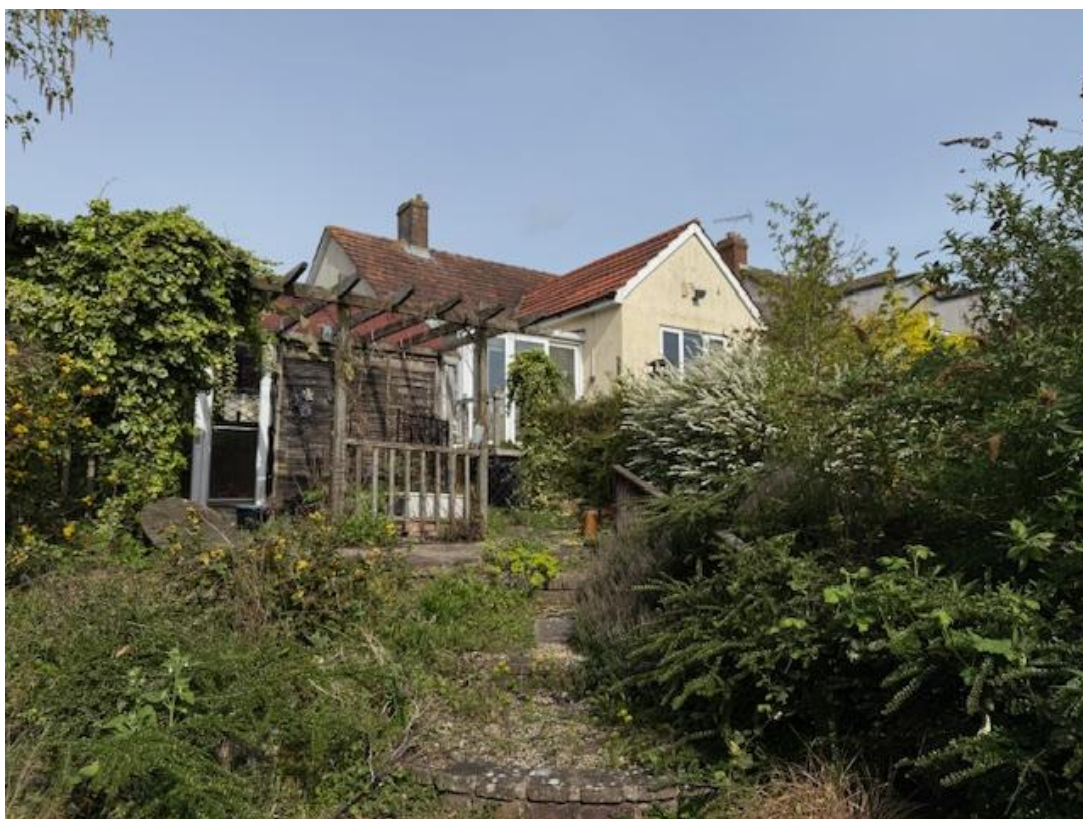
Figure 10: 5 Cambridge Road – Outbuilding & rear elevation
