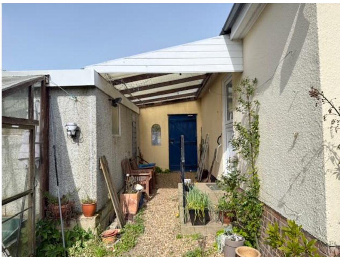
Figure 16: 5 Cambridge Road – Space between double garage and main house of 5 Cambridge Road
