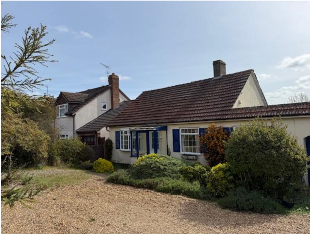
Figure 2: 5 Cambridge Road - Front Elevation & 6 Cambridge Road
