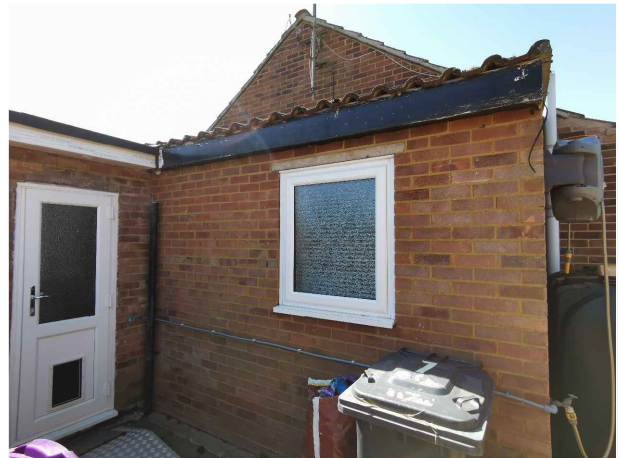
7 Willow Close - Side Extension Area to be infilled
