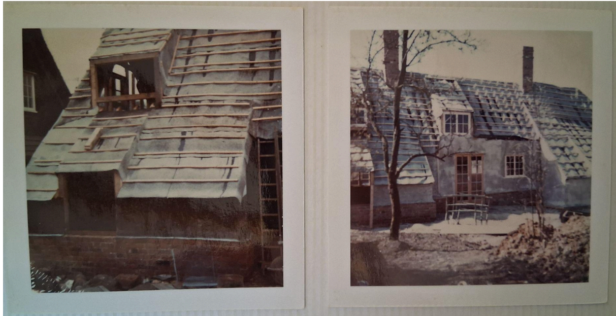
IMAGE 6: During the renovation process, circa March 1974. The new windows are installed.
