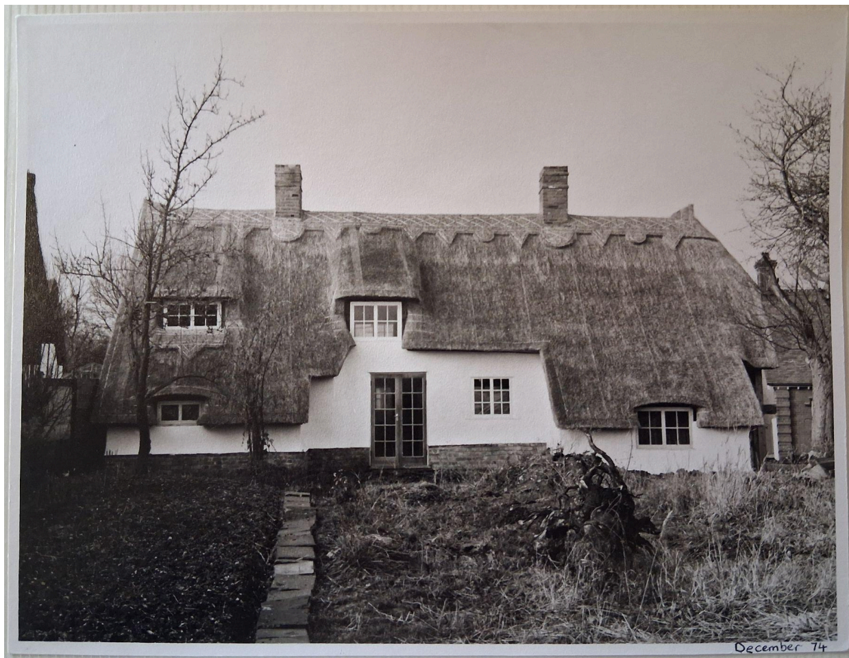
IMAGE 7: Following the completion of the renovation process, December 1974.
