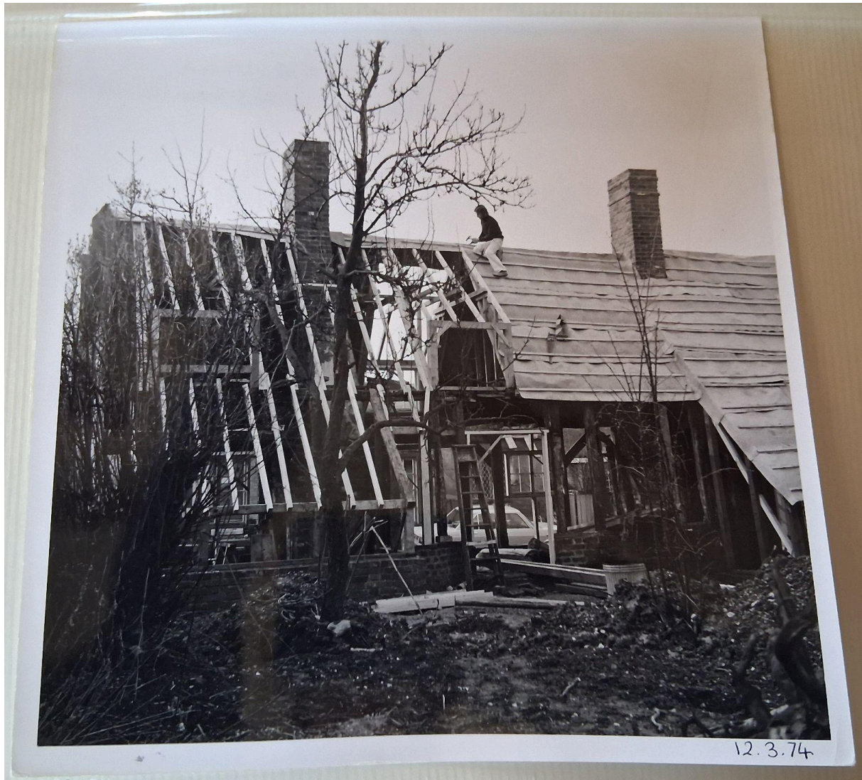
IMAGE 5: During the renovation process, 12 March 1974. The bathroom, living room and middle bedroom, seen before new windows and French doors were fitted.
