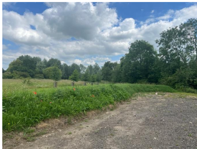
Figure 3-6 Grassed bund on site
