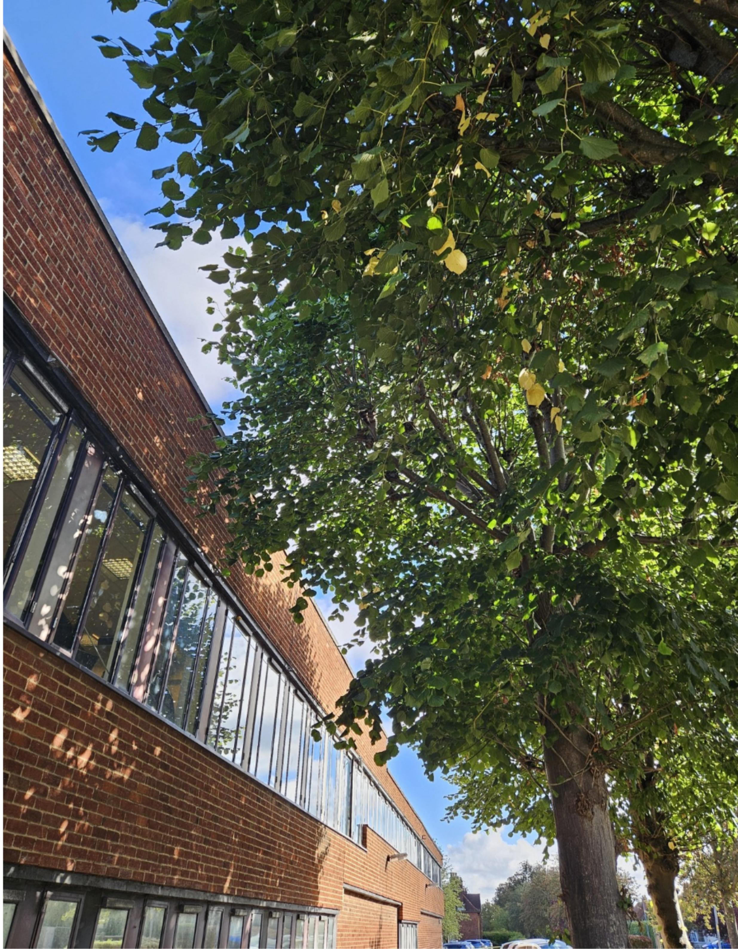
on building. Group encroaches toward the building; no significant defects noted. Repollard b
