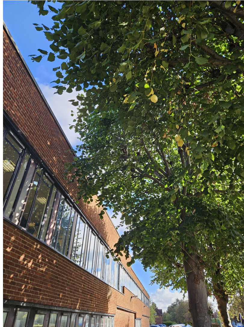
T008 - Lime x3 adjacent to the police-station building. Group encroaches toward the building; no significant defects noted. Repollard back to historic pollard points within 1 year.
