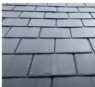
Left Slate tiles
