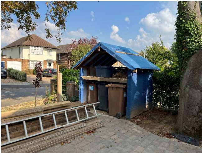
Timber frame Bin Store on the front of the property (not yet clad or tiled)
