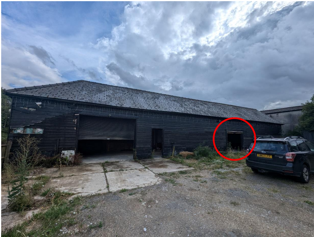
Figure 12: Location of emergence and re-entry of 3x common pipistrelle 24 th June 2025 (B2)
