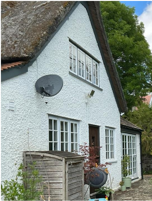
Figure 2: Exterior showing door to be removed
