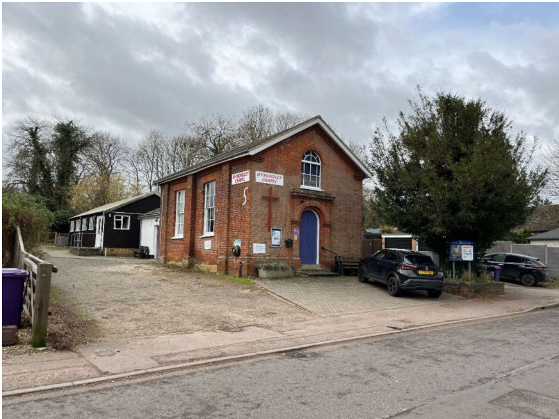
Plate 13: View of Non-designated post-medieval Baptist Chapel (Asset 199).
