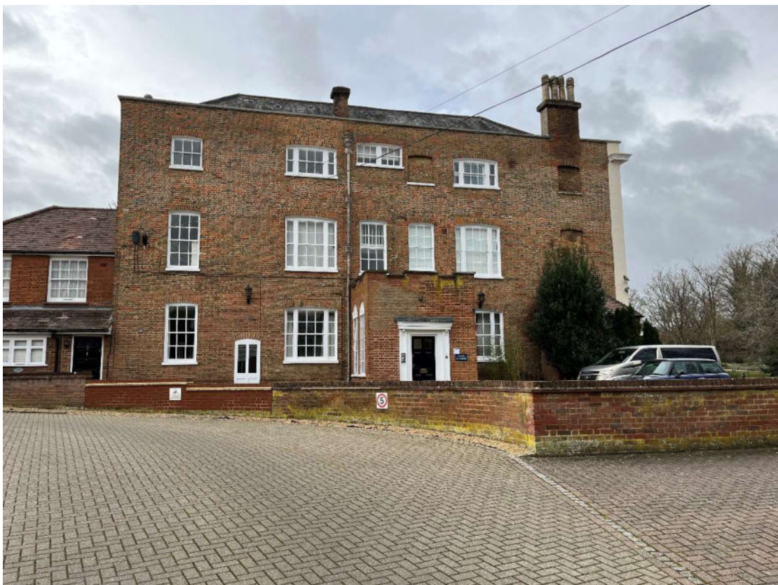
Plate 10: View of Grade II* Listed post-medieval Wymondley House (Asset 200).
