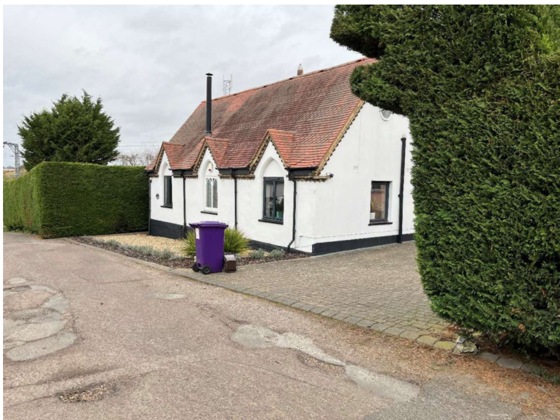
Plate 20: View of Non-designated post-medieval Old School House (Asset 83).
