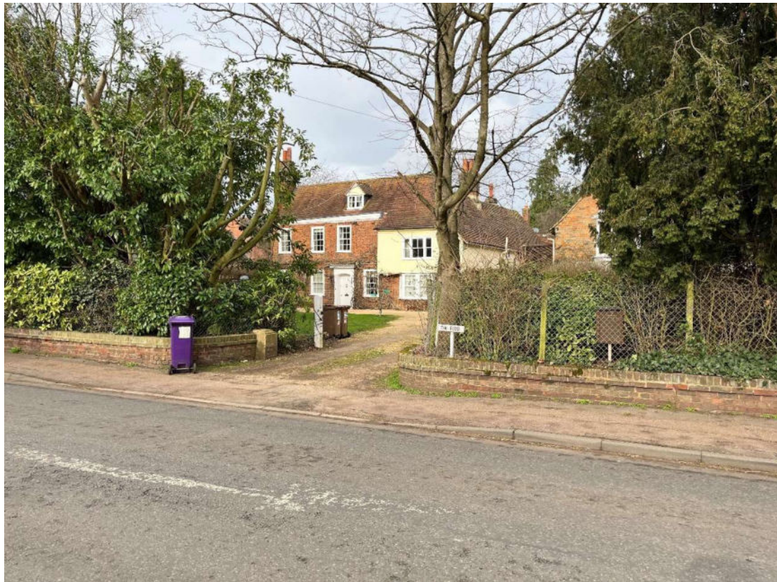
Plate 15: View of Grade II Listed post-medieval The Elms Barn and Farmhouse, converted to a single modern house (Asset 11).
