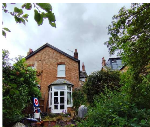
Rear Elevation Site Photograph
