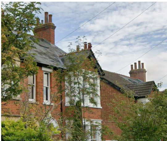
No 18 and 22 West Hill photograph - Roof lights
