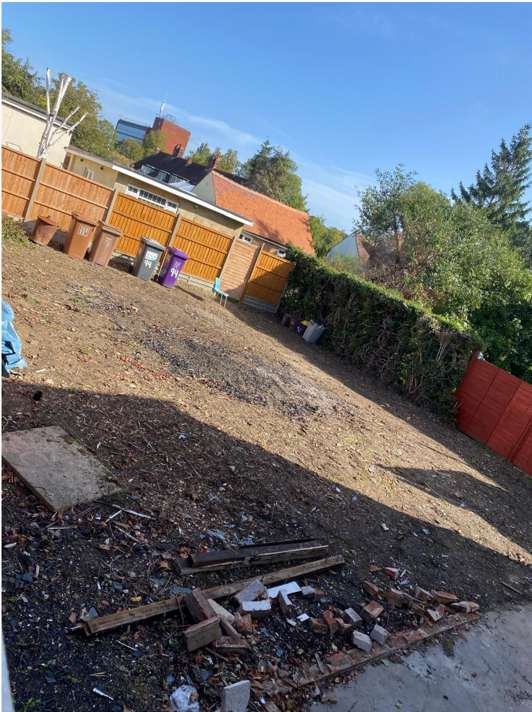
Figure A2. Rear garden area showing the outbuilding and substantial timber fencing separating the rear part of the site. The photograph also shows the extent of recent clearance.
