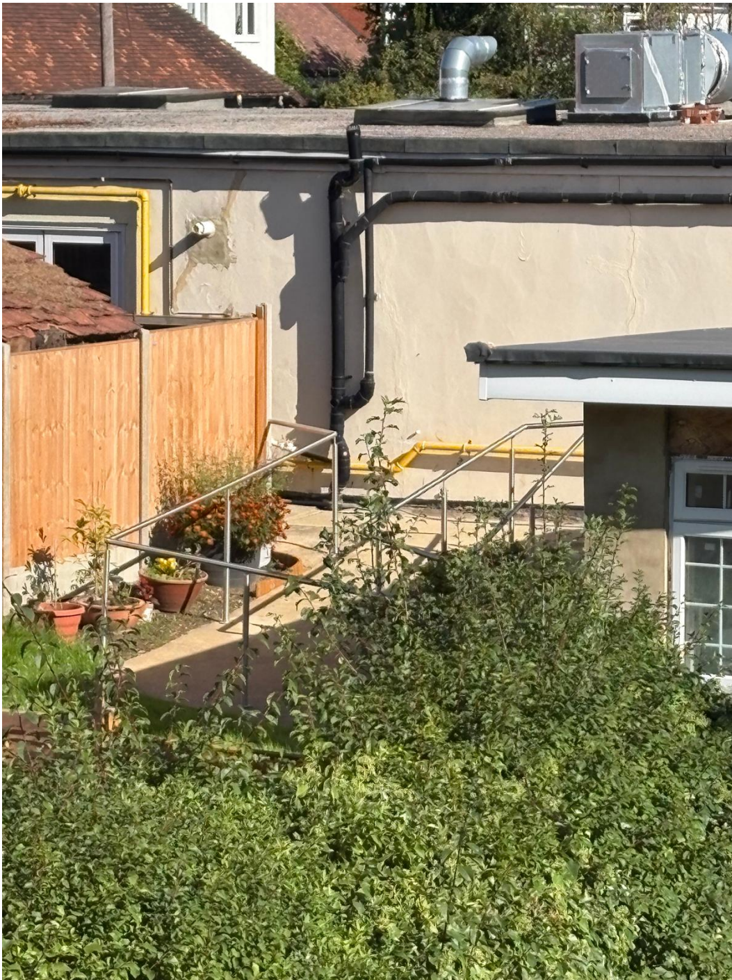
Figure A3. View towards the rear of No. 94 showing that the former rear boundary has been removed or opened and direct access established between No. 94 and the adjoining Gurdwara premises. This physical connection is relevant to understanding whether the application building is operating in association with the adjoining community and religious use.
