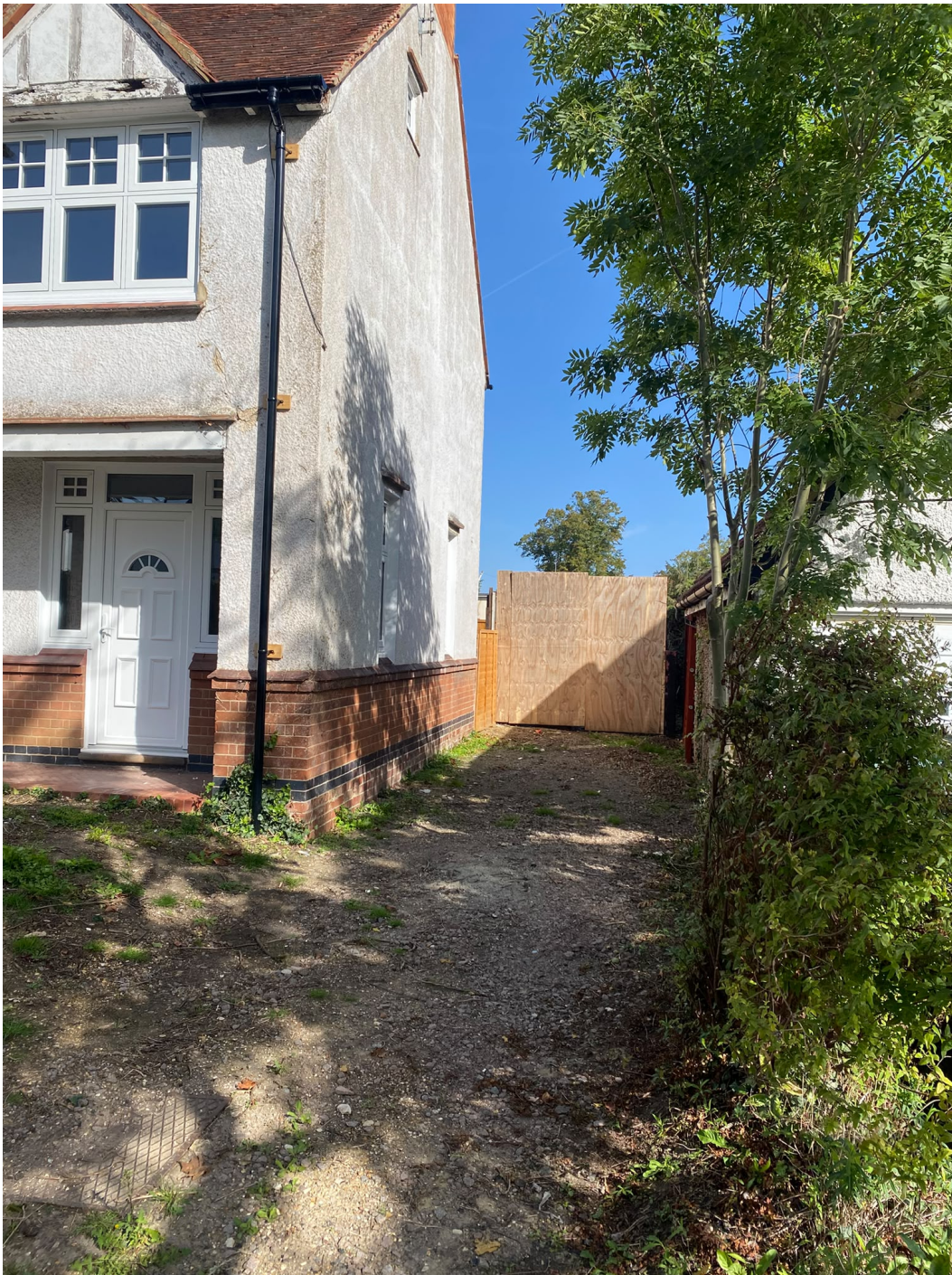
Figure A1. View beside No. 94 showing plywood hoarding/gate across the side access, restricting views towards the rear of the property.
