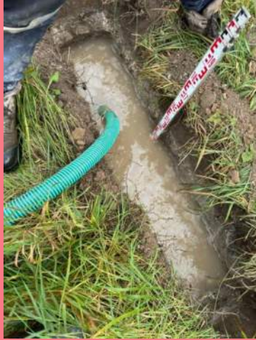
TP01 during the tests
