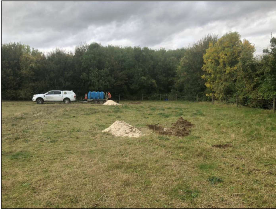
Photograph No 1 : Plant and equipment at locations of SA03 and SA04
