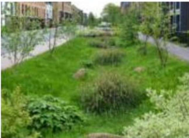
SuDS used to enhance streets
