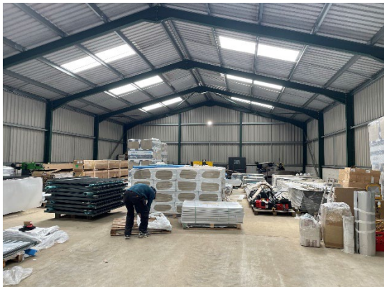
Photo 9. Interior of modern shed (B2)
