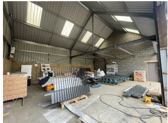
Photo 10. Interior of modern shed (B1).
