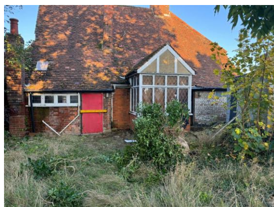
Views of plot from front, side lane, garage face and rear cat slide
