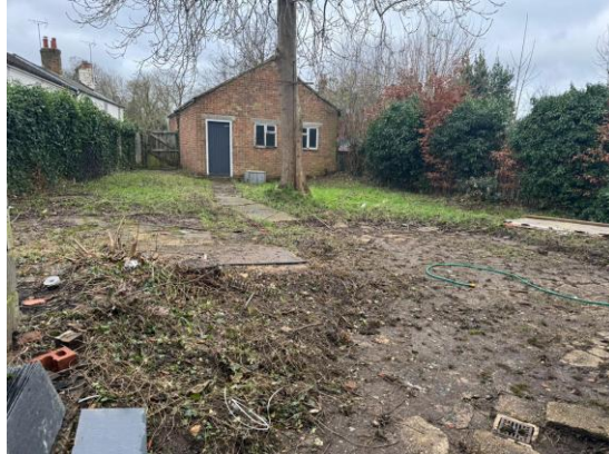
Views of the storage block and of the garage from the garden
