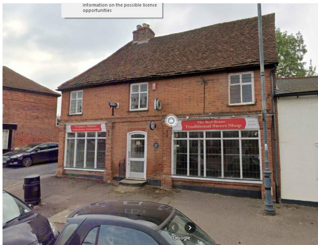
Photograph of existing building showing existing signage features
