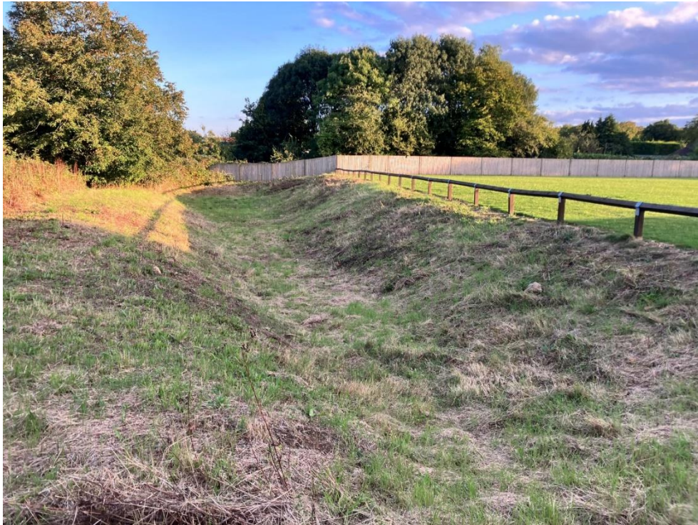
Photograph 6 - the swale on the east boundary of the affected area of playing field
