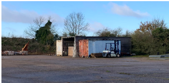
Fig 1.3.1 // Existing storage structures
