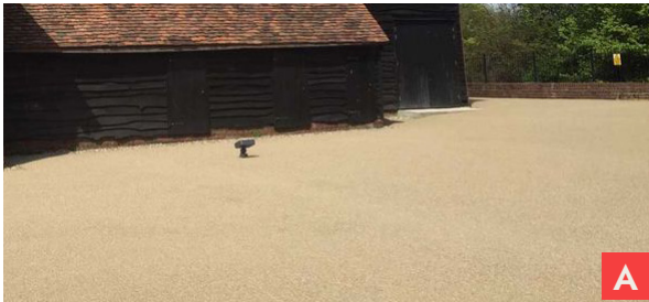
Fig 3.3.1 // Permeable bonded gravel courtyard
