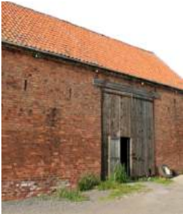
Example of Historic Barn with vertical ventilation slots
