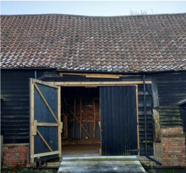
Existing Barn Brick Bonds
