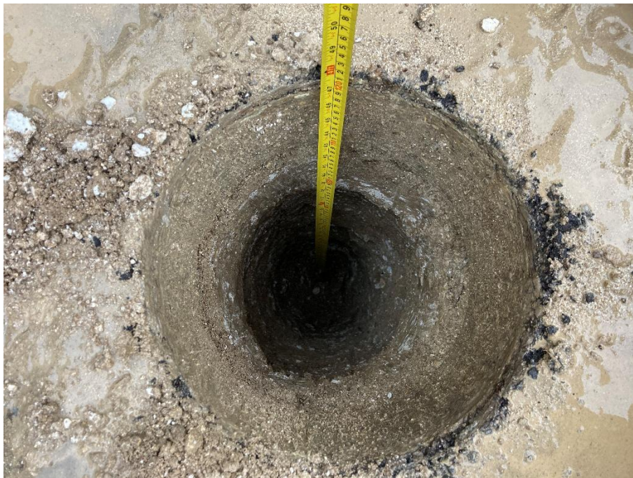
P6: Photograph showing inspection pit from BH01
