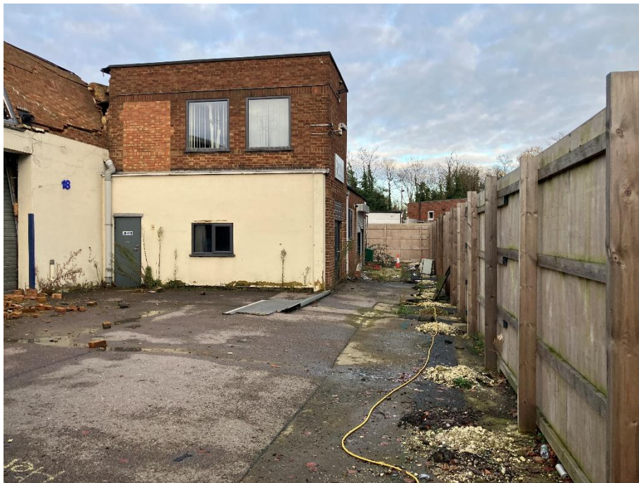
P4: Photograph showing northeastern corner of the site
