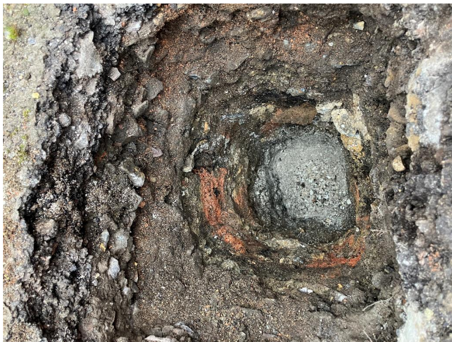
P40: Photograph showing inspection pit from BH04
