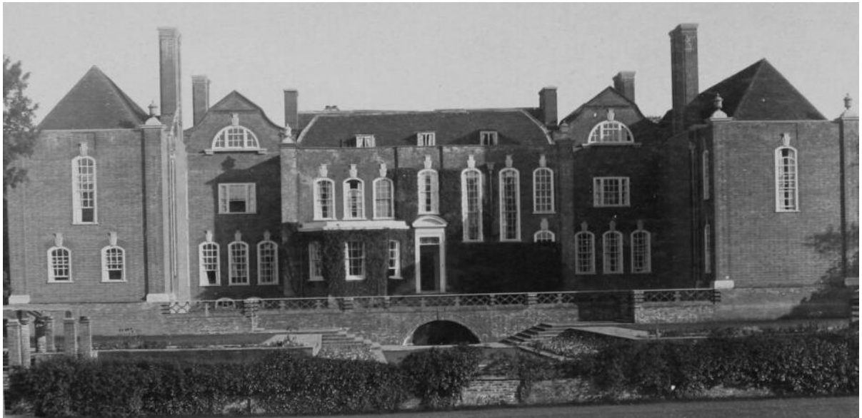
North Elevation of Lutyens' West Wing which shows us there was a single window on the north Elevation of the West wing.
