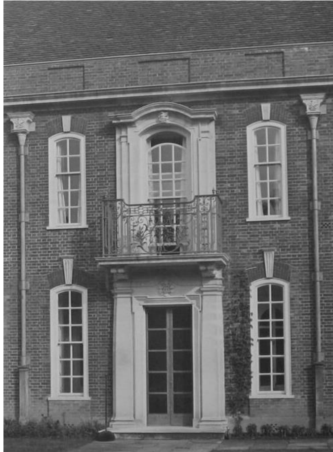
West Elevation of Lutyens' West Wing.
