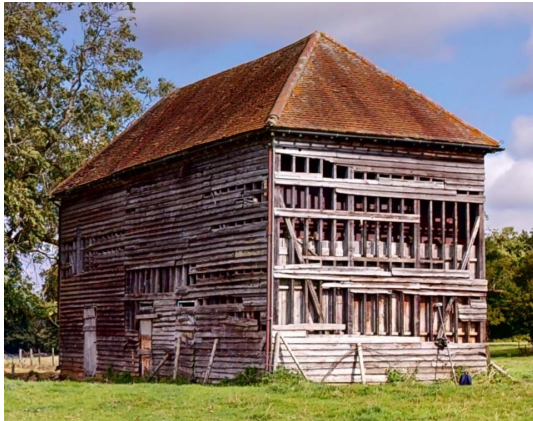
Looking North East
