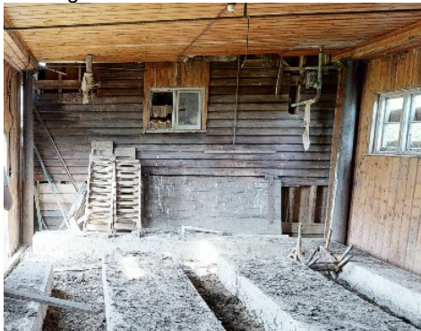
Internal Wall (Original South Elevation)
