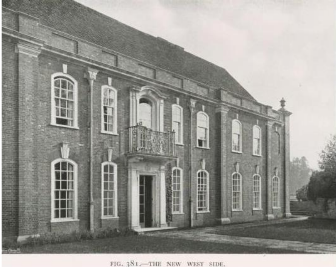
West Elevation of Lutyens' West Wing prior to the roof being raised.
