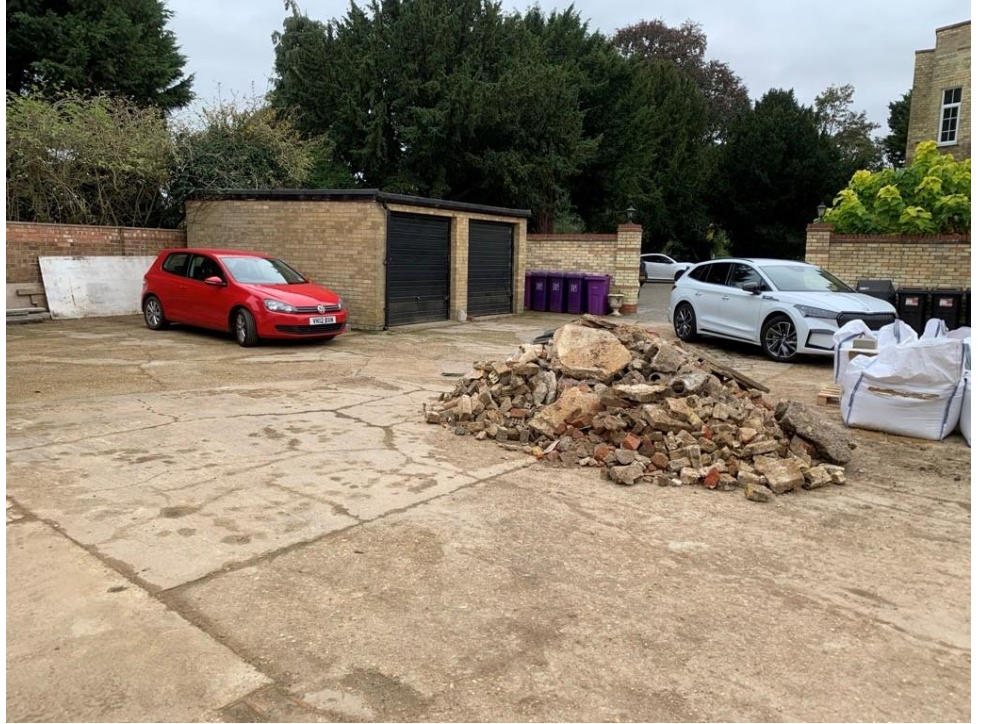
The walled concrete yard, double garage and existing vehicle access
