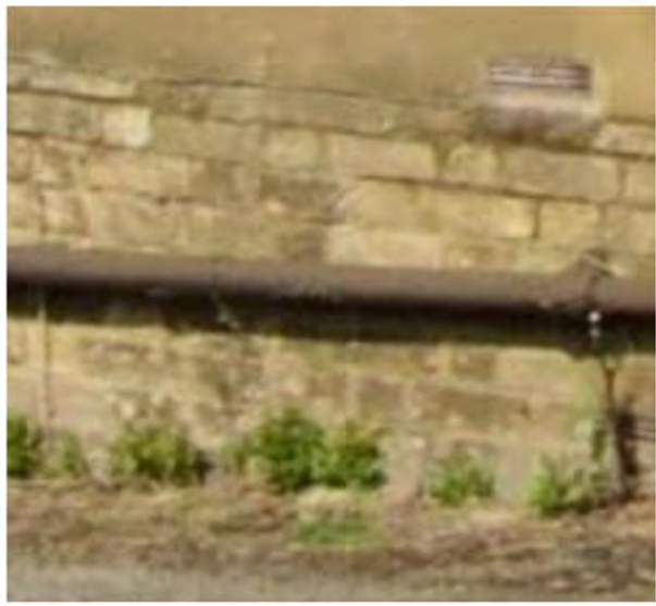
Facing Brickwork: (buff)
