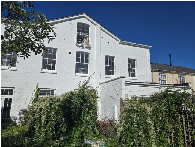
Walls painted white to match host building
