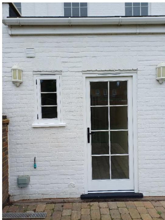
Rear wc window & rear entrance
