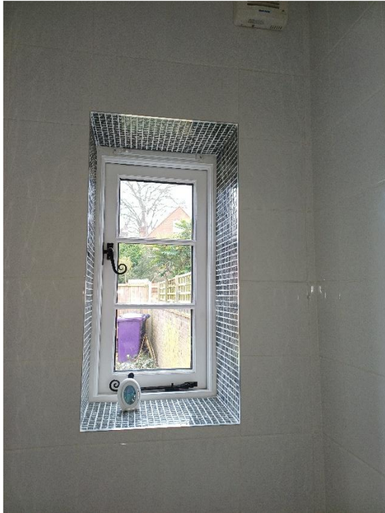
New timber window viewed from wc
